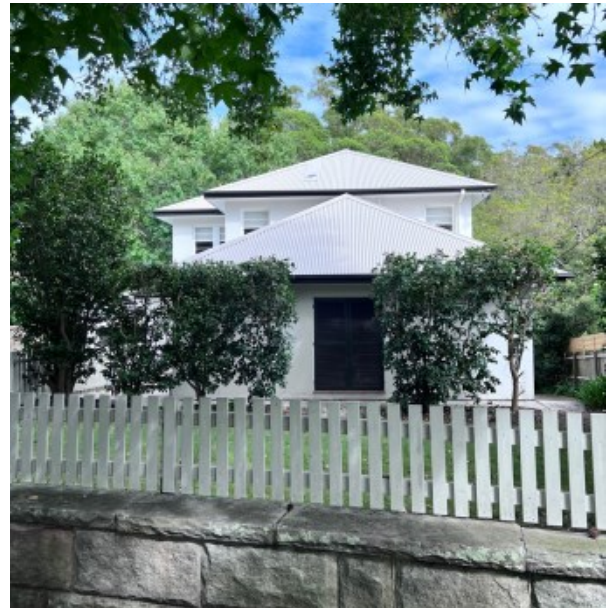
After: Colorbond roof and external painting
