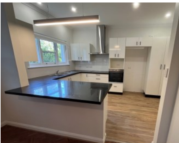
Completed new kitchen
